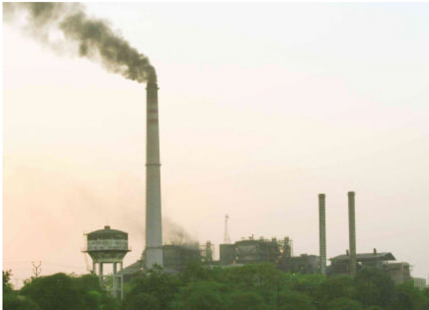
Panki Power House
